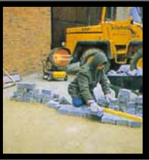
Winter construction: heats up materials, machines, and working sites
